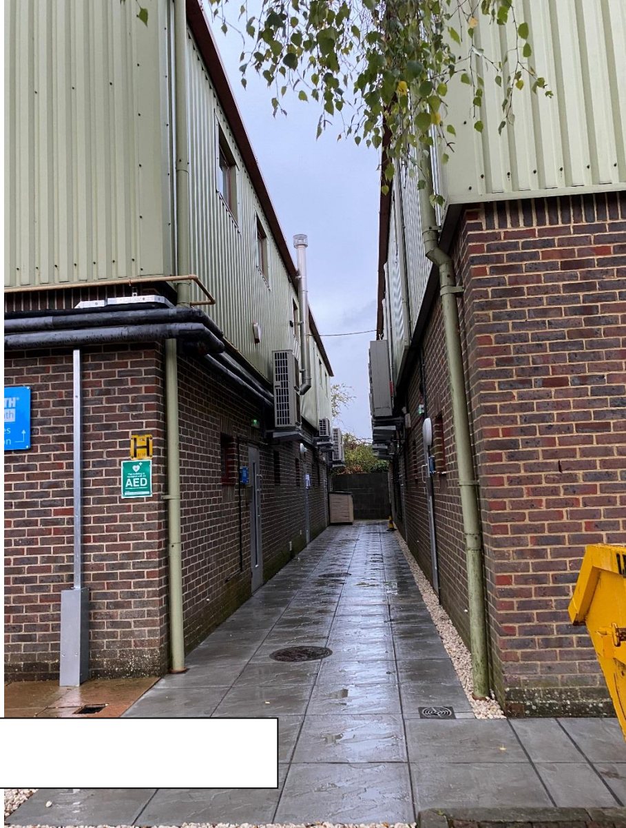
Gap between the two units
